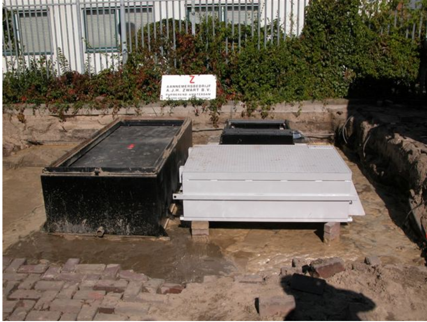
Figure 2.5.: Previous prototype of the underground substation. Transformer case left, MV-compartment upper right, LV-compartment lower right (grey). Picture from Liander archives.
