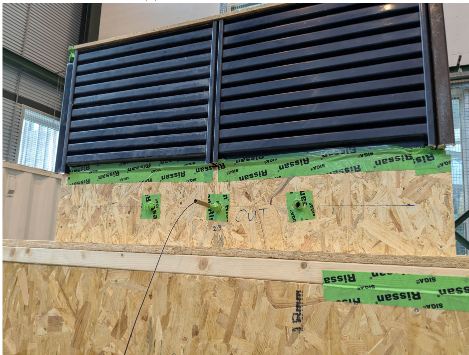
(b) Flow Locations Vault 1 Outlet
