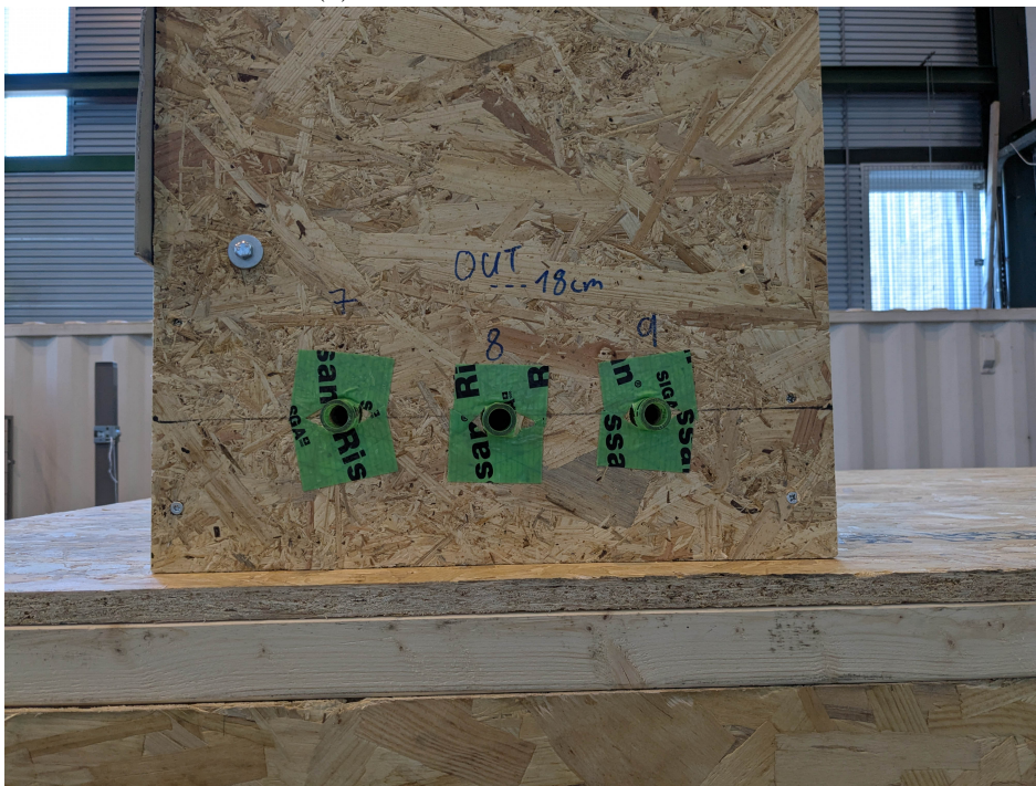
(b) Flow Locations Vault 2 Outlet
